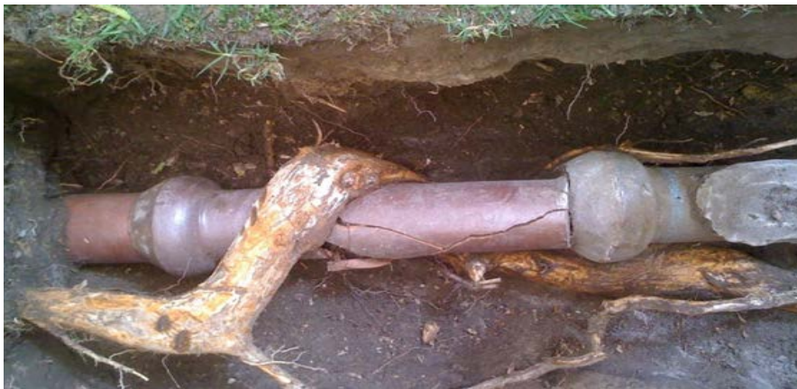
Photo 3 shows a tree root wrapping around a sewer pipe and squeezing it to the point of collapse.
