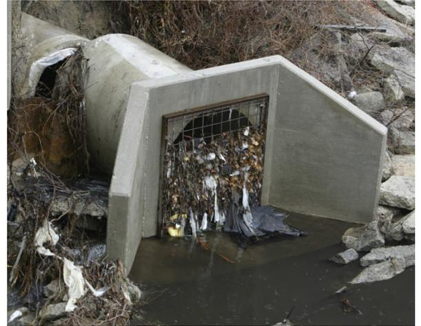
*Clogged storm water outlets and broken pipes and structures create pollute the streams and reduce water quality.*
