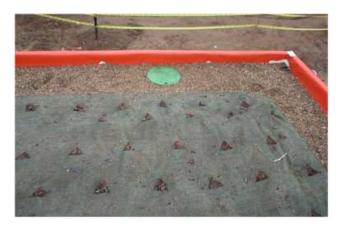
These assemblies are suitable for roofs with pitches less than, or equal to, 1.5:12. Large vegetated covers will generally incorporate a network of perforated internal drainage conduit.
