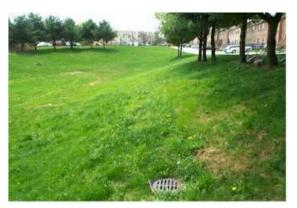
An Infiltration Trench is a "leaky" pipe in a stone filled trench with a level bottom. An Infiltration Trench may be used as part of a larger storm sewer system, such as a relatively flat section of storm sewer, or it may serve as a portion of a stormwater system for a small area, such as a portion of a roof or a single catch basin. In all cases, an Infiltration Trench should be designed with a positive overflow.
