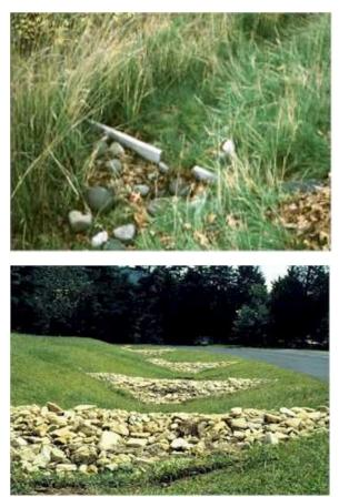
check-dam, a better approach might be to allow low flows (2-year storm) to drain through the stone, while allowing higher flows (10-year storm) drain through a weir in the center of the dam. Flows through a stone check-dam are a function of stone size, flow depth, flow width, and flow path length through the dam. The following equation can be used to estimate the flow through a stone check dam up to 6 feet long:
