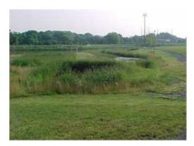
Constructed Wetlands are shallow marsh systems planted with emergent vegetation that are designed to treat stormwater runoff.
