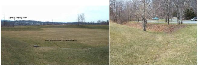
Figure 9-12. Level spreader distributes stormwater into the infiltration basin.
