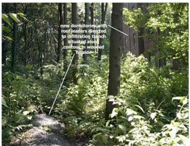
Figure 9-27. Level spreader pipe/infiltration trench in woods.
