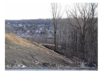
Figure 5.1-4. Steep slope development with woodland removal.
