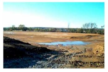
Soil amendment and restoration is the process of improving disturbed soils and low organic soils by restoring soil porosity and/or adding a soil amendment, such as compost, for the purpose of reestablishing the soil's long-term capacity for infiltration and pollution removal.
