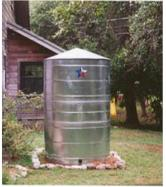
**Rain barrels** – barrel (or large container) that collect drainage from roof leaders and store water until needed for irrigation.
