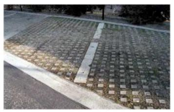
Figure 5.10-2 Overflow parking using permeable pavers
