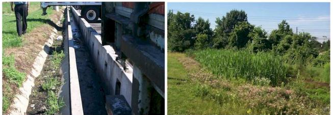
Figure 9-16. Perimeter trench drain.
