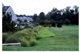
Identify, protect, and utilize the site's natural drainage features as part of the stormwater management system.
