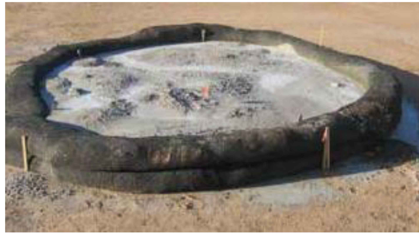
FIGURE 3.18 Typical Compost Sock Washout Installation
