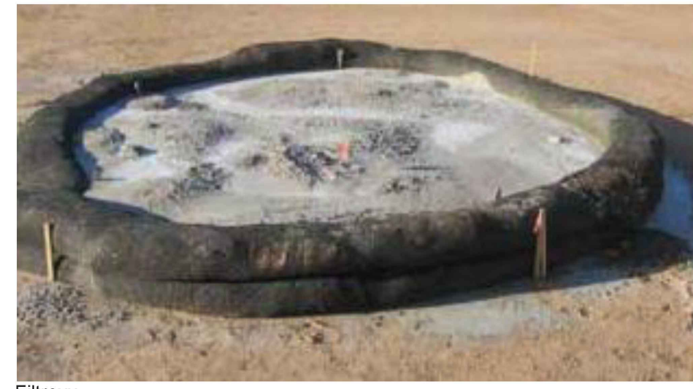
FIGURE 3.18 Typical Compost Sock Washout Installation
