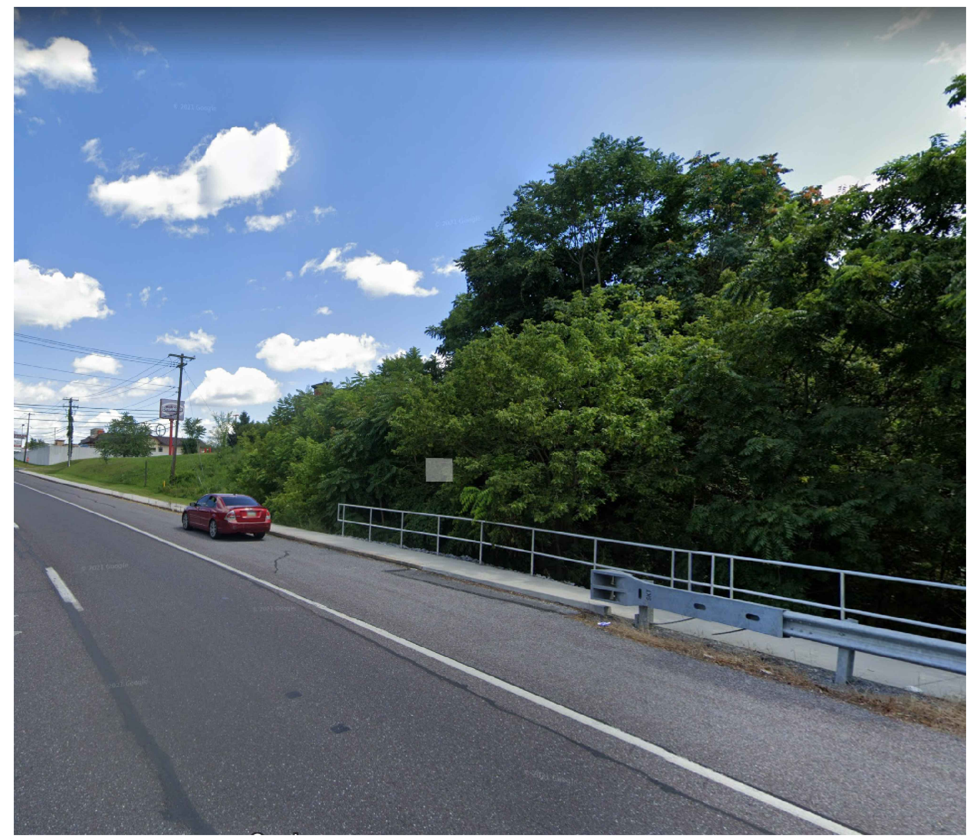
① EXISTING STREET VIEW
