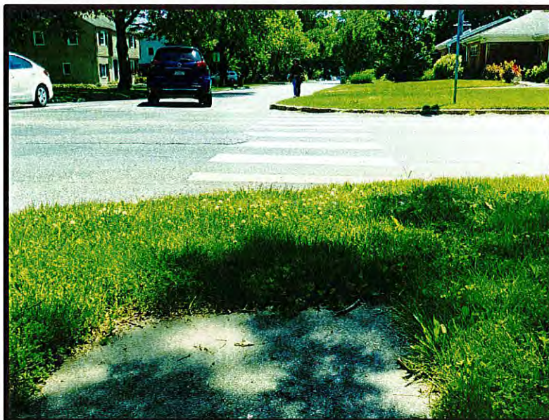
Figure 2: EB Schoolhouse Lane Sidewalk Gap
