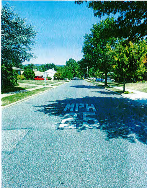
500 Blk Shield St facing N/B "25MPH" Sign
