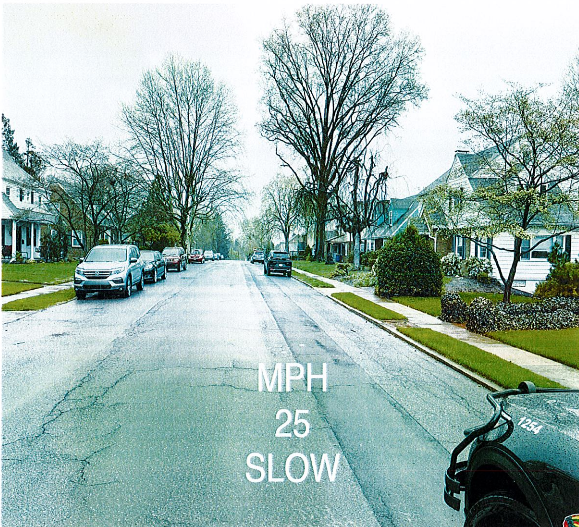
Looking East in the 3100 Block of Schoolhouse Lane
