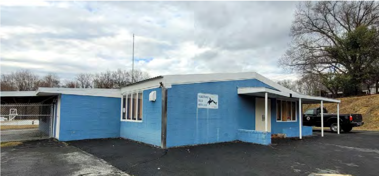
Southeast Side of the Pool Clubhouse and Locker Rooms
