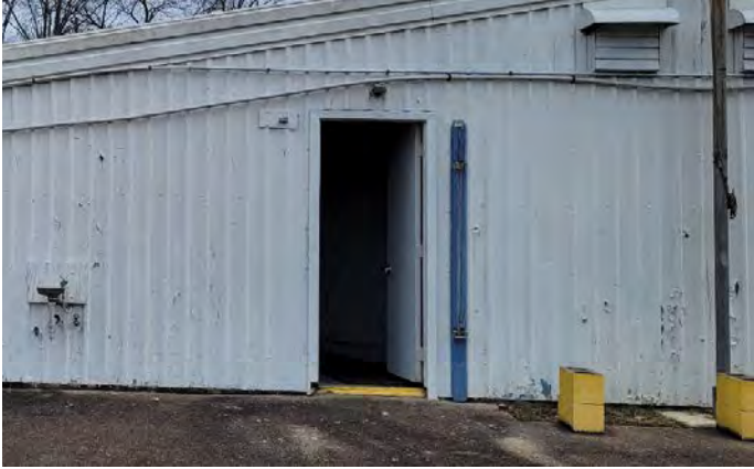
Metal Cladding on the West Elevation
