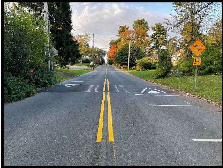
Figure 9: Signs and pavement markings
