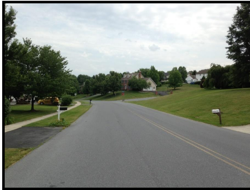
Figure 13: Wide streets with no curbs or parked vehicles will have higher speeds
