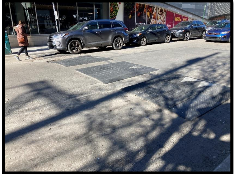
Figure 19: Temporary speed cushions, Philadelphia
