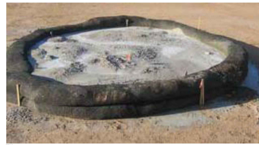
FIGURE 3.18 Typical Compost Sock Washout Installation
