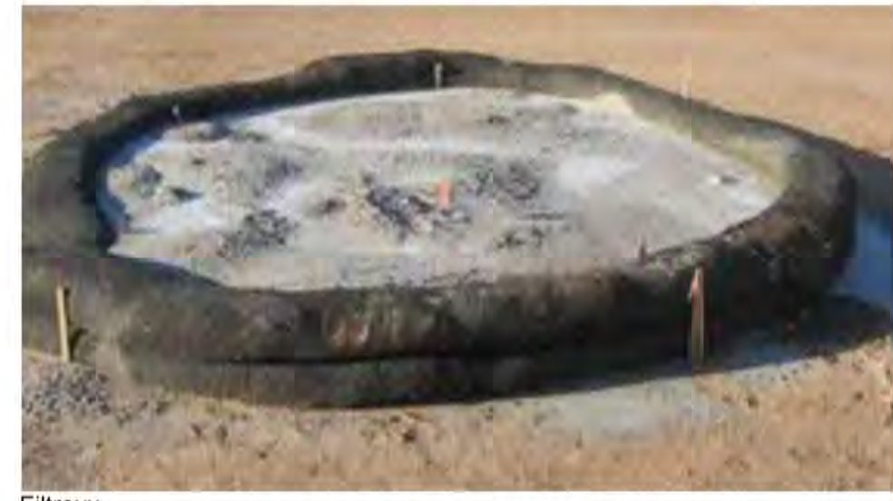
FIGURE 3.18 Typical Compost Sock Washout Installation
